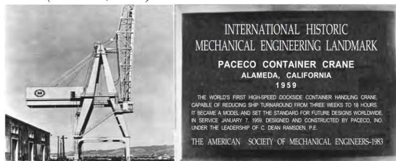
Figure 2.7 The first container crane (*ASME-b, 1983*)
