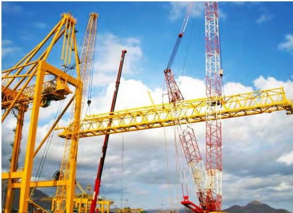
Figure A-1 Derrick boom being lifted into place
